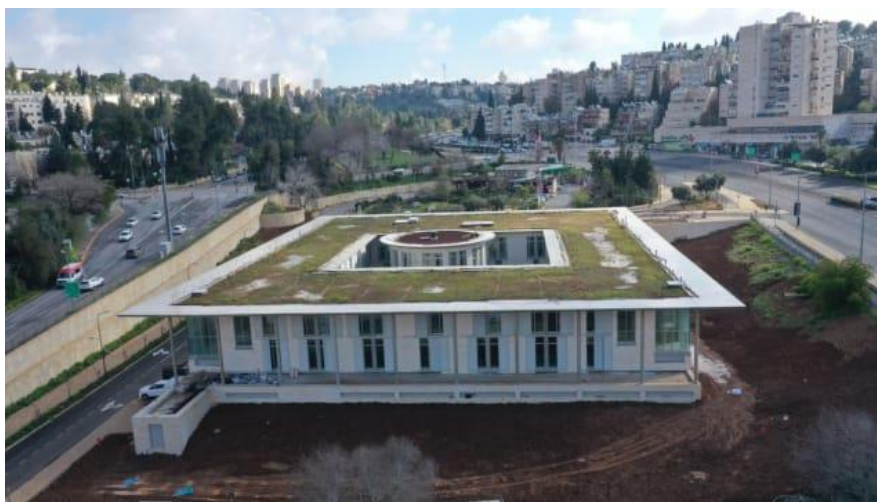
The Mandel Building, adjacent to the Botanical Garden in Jerusalem, which was to have been dedicated in the coming weeks. It has the largest green roof in Israel. Amir Balaban / Yehidat
